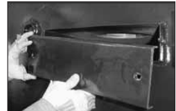
Removing Flue Cover
