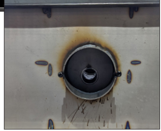
Combustion Air Tube (Behind Front Fan)
