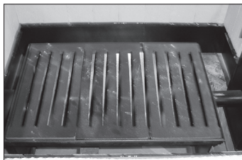
Ash Pan (below grates)
