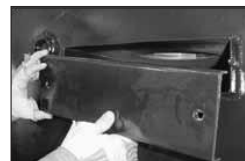
Removing Flue Cover
