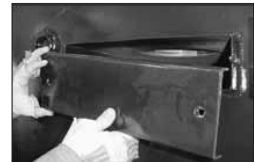
Removing Flue Cover
