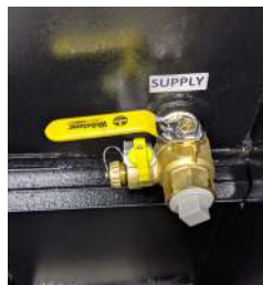
Supply Valve (closed)
