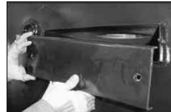
Removing Flue Cover
