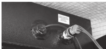
Water Level Probe
