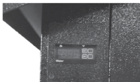
Electronic Aquastat Controller
