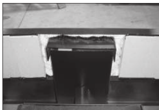
Air tube holds the air restrictor.
