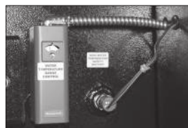
Water Temperature Range Control
