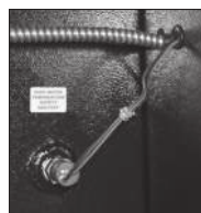
High Temp Safety Shutoff
