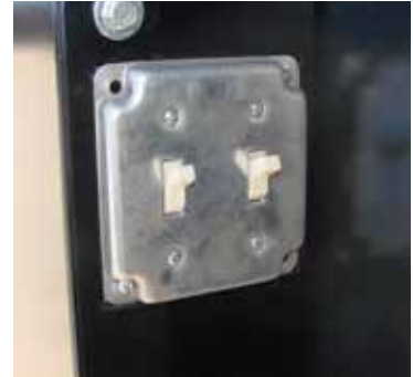
Ignitor Switch (right switch)
