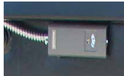
High Water Temperature Safety Shutoff Control
