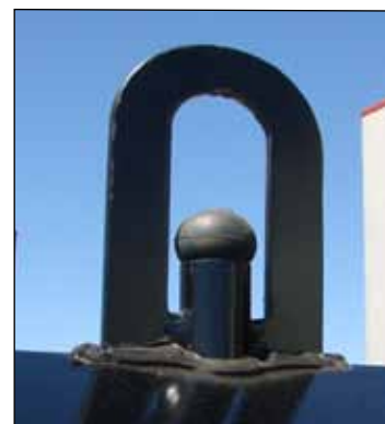
Relief Vent Pipe and Weighted Pop Off Ball
