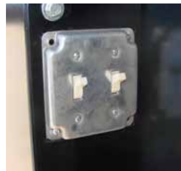
Front Light and Fan Power Switch (left switch)
