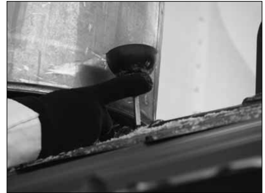
Relief Vent Pipe and Weighted Pop Off Ball
