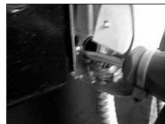
Removal of Aquastat Cover
