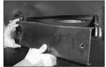
Removing Flue Cover
